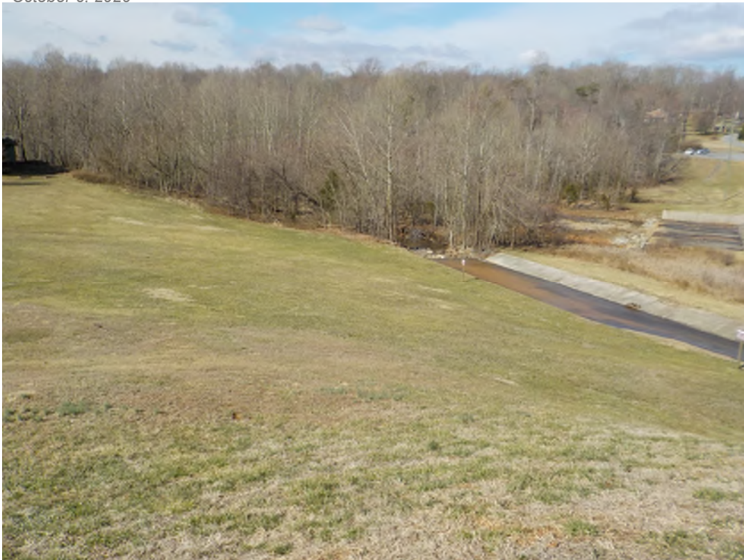
Photograph 3: Sediment disposal area (to left), and concrete dam spillway (to right)
